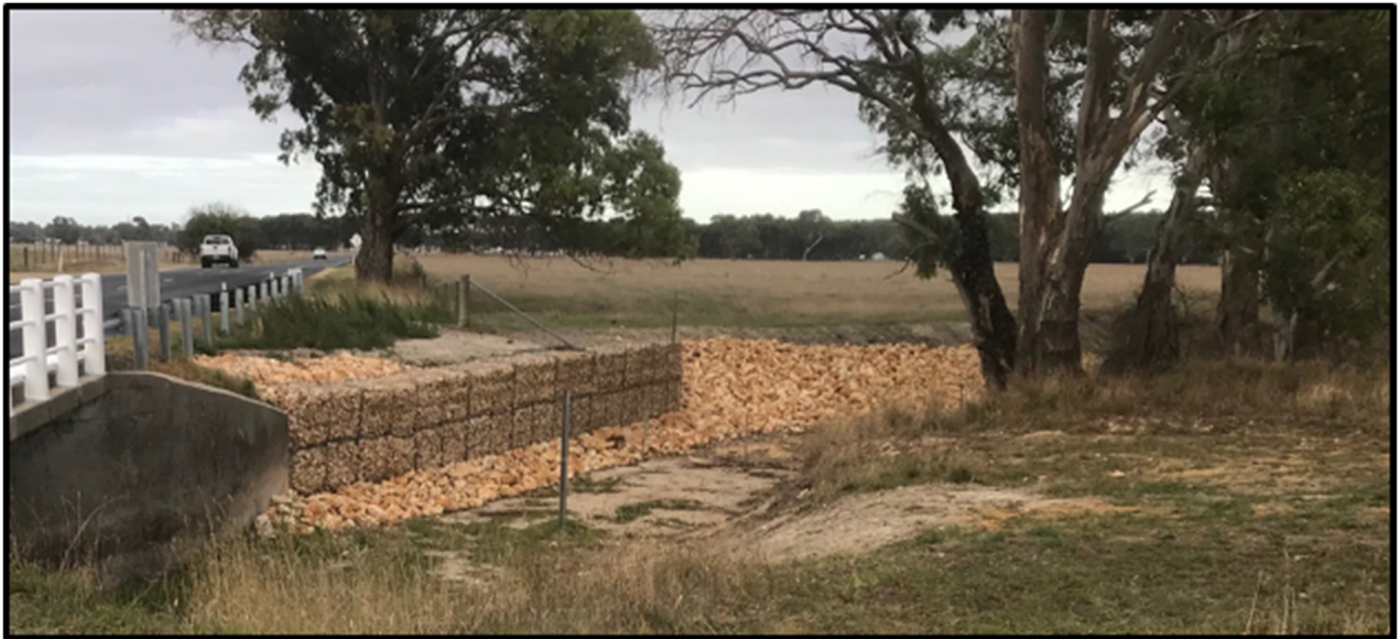
Cadgee Road Bridge, Wild Dog Valley - Stabilisation
