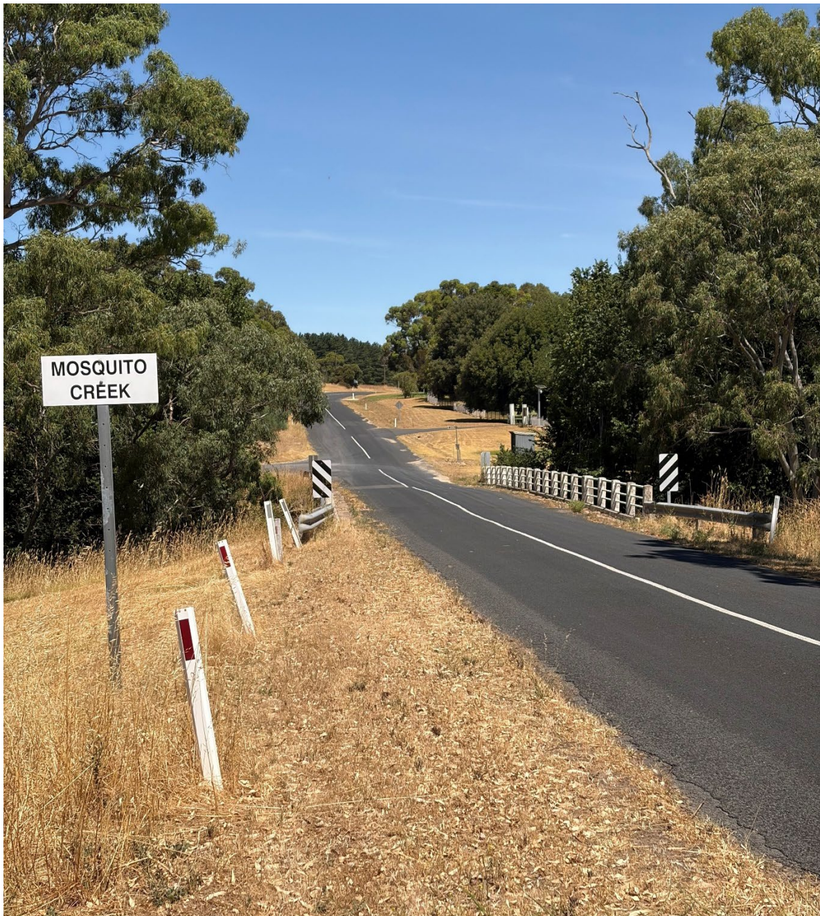
Struan House Road Bridge
