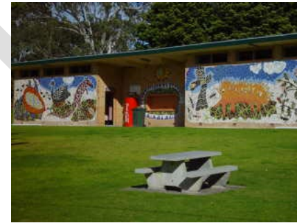
Toilets and change rooms
